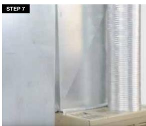
7. Prepare the duct (return or supply) for installation. Evaluate the ideal area for installing the air purifier. The reflection chamber should always be parallel\* to the airflow. Ensure that the purifier will fit into the plenum and position it keeping in mind to minimize plastic exposure to direct UV light.
