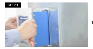
1. Take the SR Max out from the ductwork by removing the 4 screws located on the cover (4 corners) that hold it to the frame
