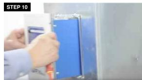
10. Finalize the SR Max installation in the duct by placing the unit into the frame, guided with the alignment pins.
