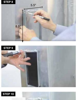
8. Use the included metal frame to trace the outline onto the duct. Allow for a 1/8" space around the marking as to allow the frame to sit properly in the duct. The duct opening window should have the following dimensions: 8.5" x 5.5".
